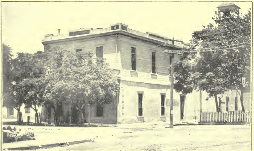
TUCSON CITY HALL.
